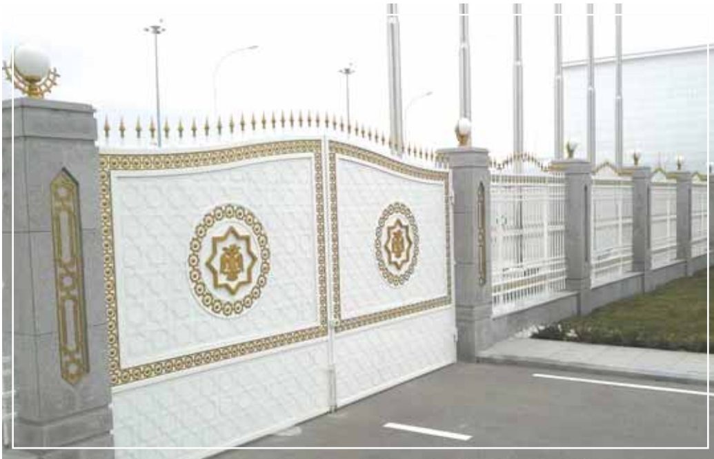
International Airport. Ashgabat / Turkmenistan
