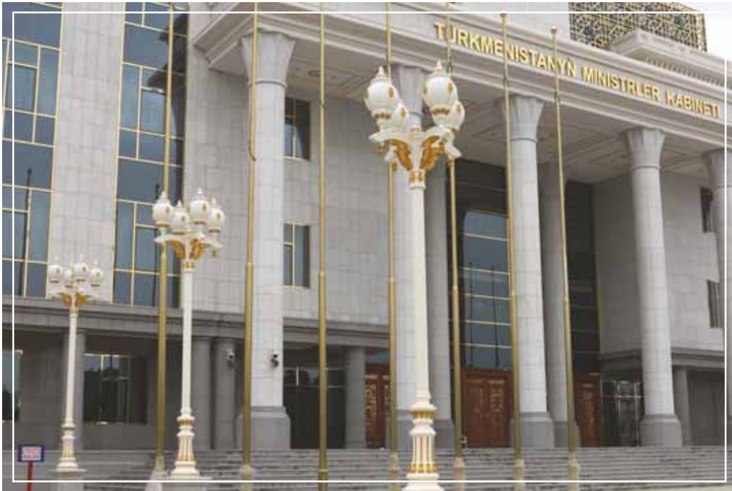
Ministry Buildings. Ashgabat / Turkmenistan
